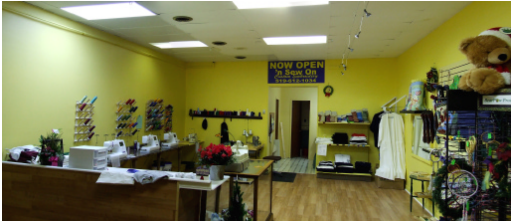
BEFORE: Retail store lit with existing fluorescent troffer lights and halogen track-lights
