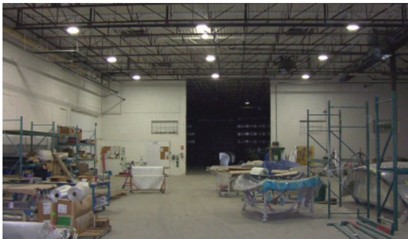
AFTER: Nine of the induction lamp 200W highbay light fixtures can be seen in this photo.
