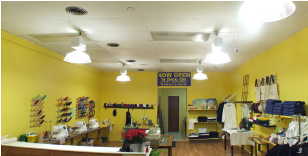
AFTER: Retail store lit with Magnetic Induction Lowbay fixtures and LED track-lights after lighting renovations.
