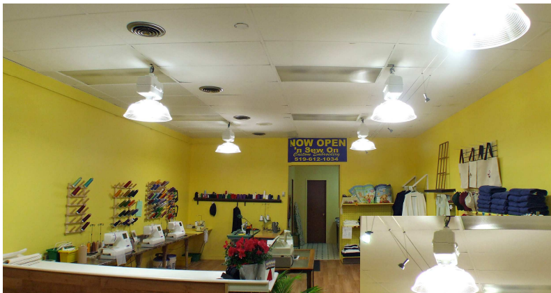
Left: N' Sew On - Retail store lit with GreenTech Induction and LED lights after lighting renovations (looking from the front door - the sixth fixture is not visible due to its placement for lighting the store window).
