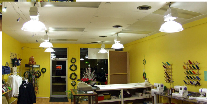
Right: N' Sew On - Retail store lit with GreenTech Induction and LED lights after lighting renovations (looking from the back towards the front door - the folding display wall at the front right is in the "store closed" position).
